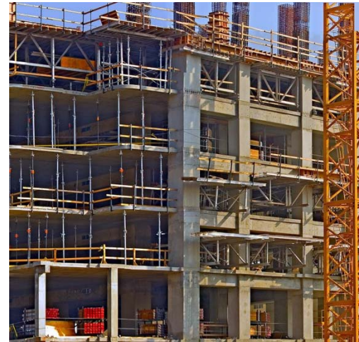
Firm building structure
